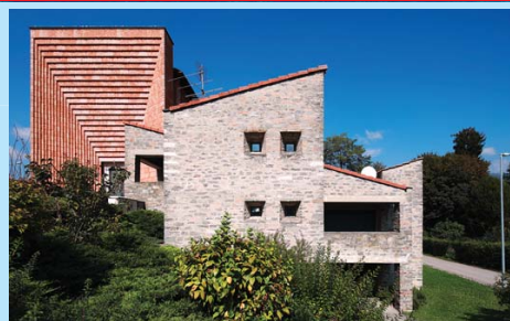
The first construction of Mario Botta was this parish house in Genestrerio, half way between Mendrisio and Stabio, 1961–63.
